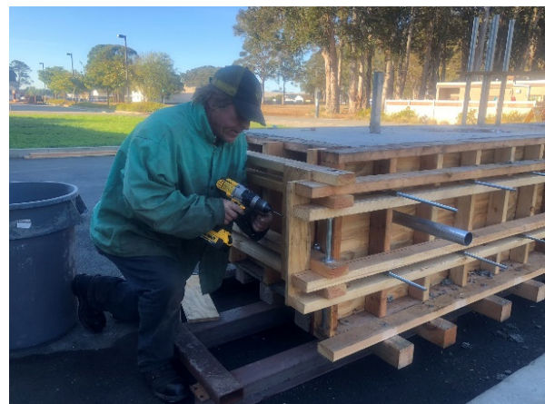
Figure B.10 Remove the formwork.
