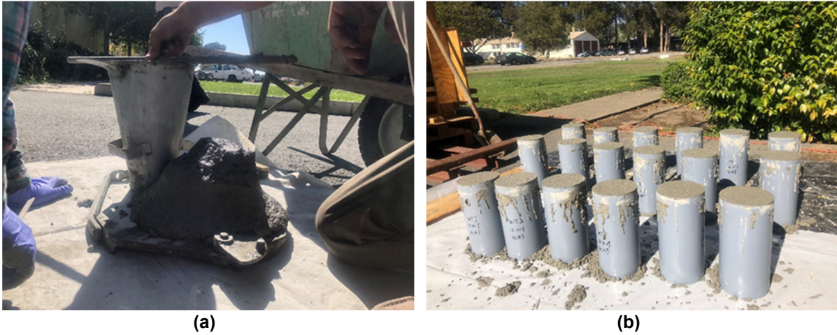
Figure 6.26 (a) Slump test; (b) sample concrete cylinders for material testing (cap beam and foundation).
