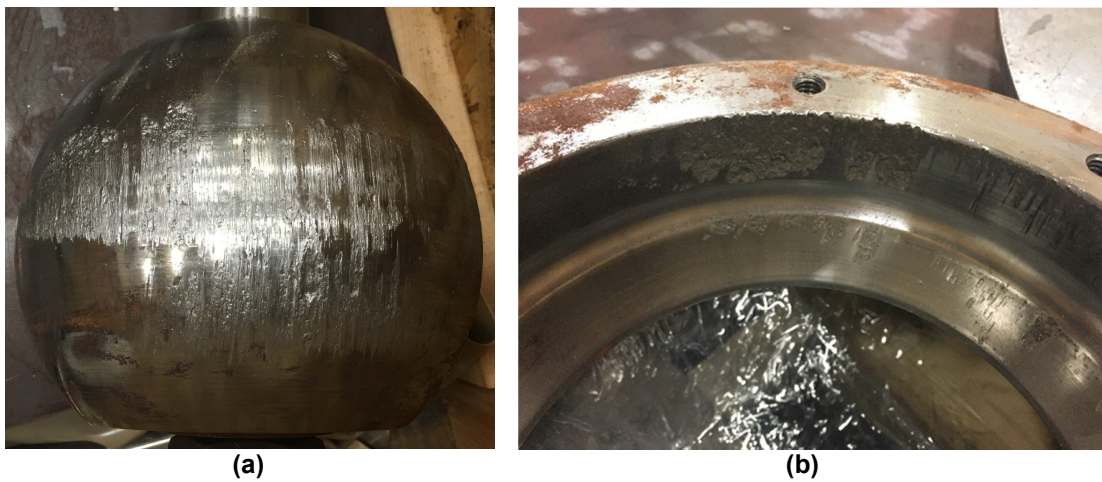
Figure 5.17 Damage conditions of the different V-connector components: (a) ball hinge; (b) hinge holder.
