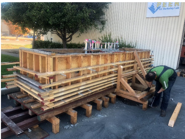
Figure B.10 Remove the formwork.
