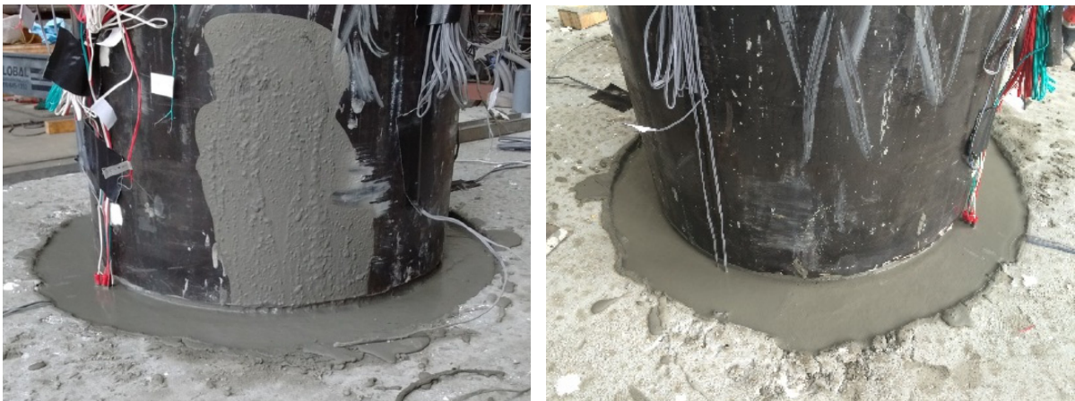
Figure C.5 Foundation sockets grouting.
