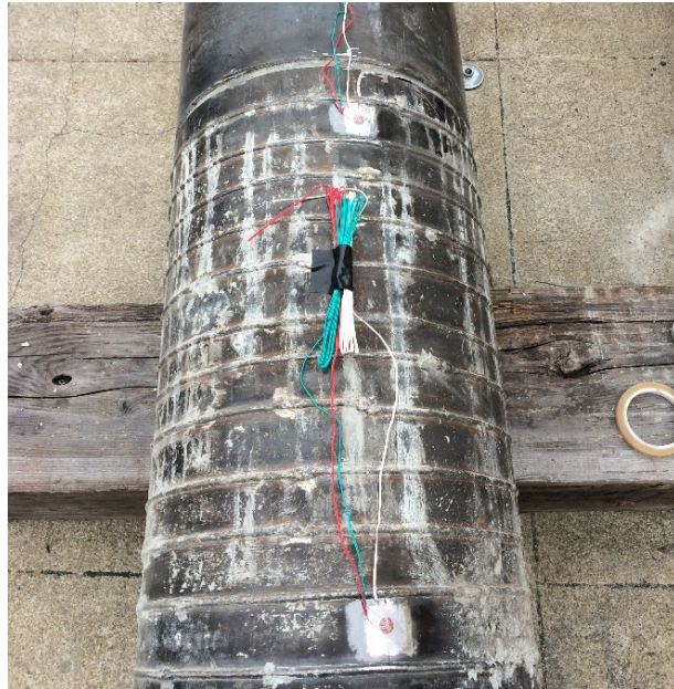
Figure 6.39 Rosette strain gauges on the steel shell.
