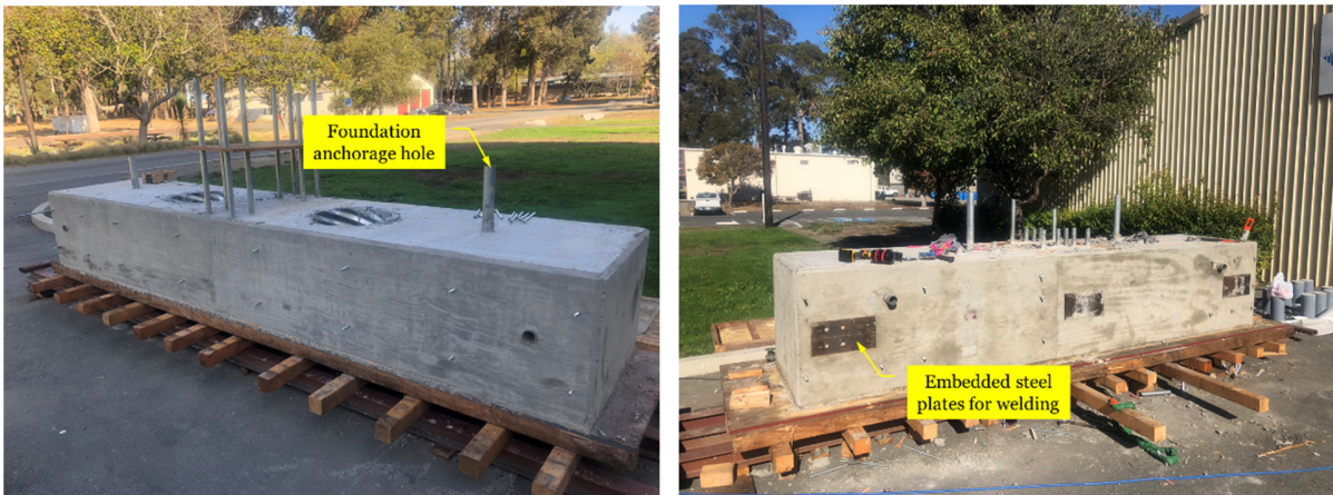
Figure 6.19 Final completed foundation (left) and cap beam (right).
