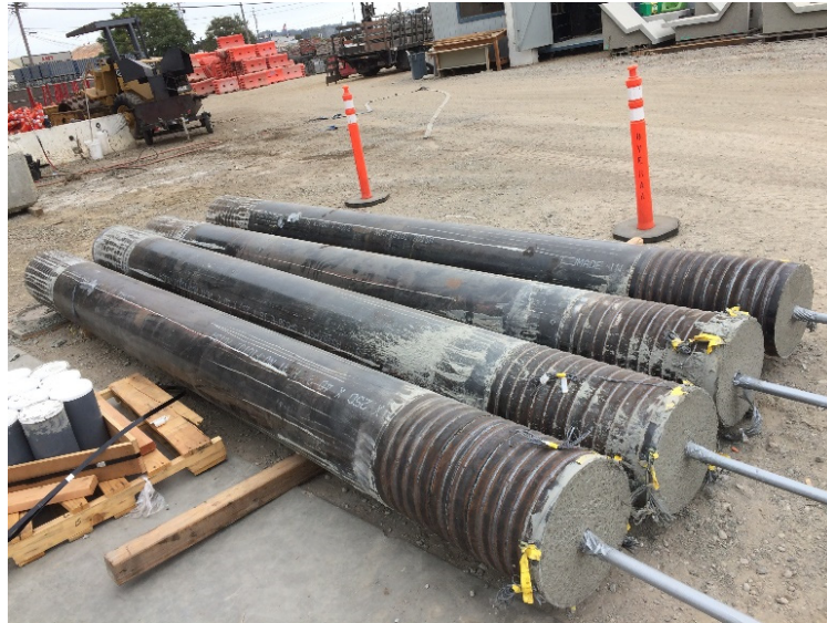
Figure 6.16 Final completed columns.
