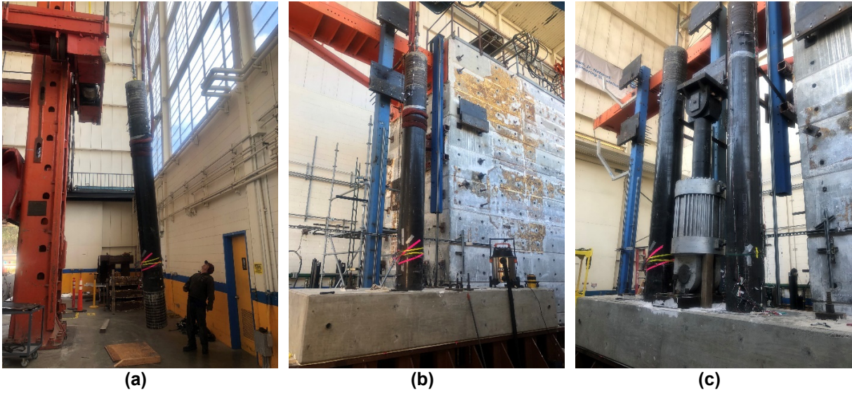
Figure C.4 (a) Pick up the column; (b) install and level the column; and (c) install the vertical actuator between the two columns.
