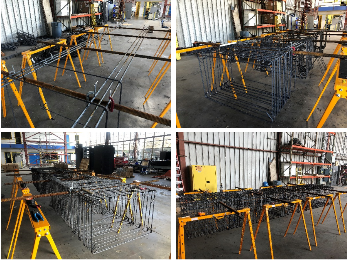
Figure B.6 Different stages of foundation reinforcing bar cage construction.
