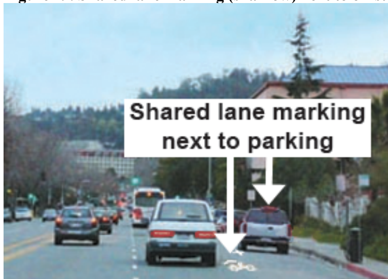
Figure 29. Shared lane marking (sharrow) next to on-street parking
