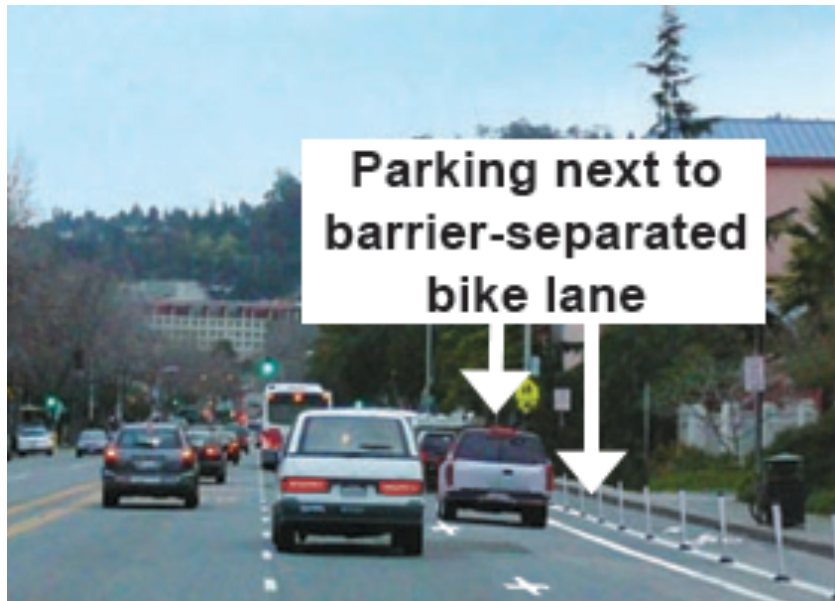
Figure 26. Barrier-separated bike lane next to on-street parking
