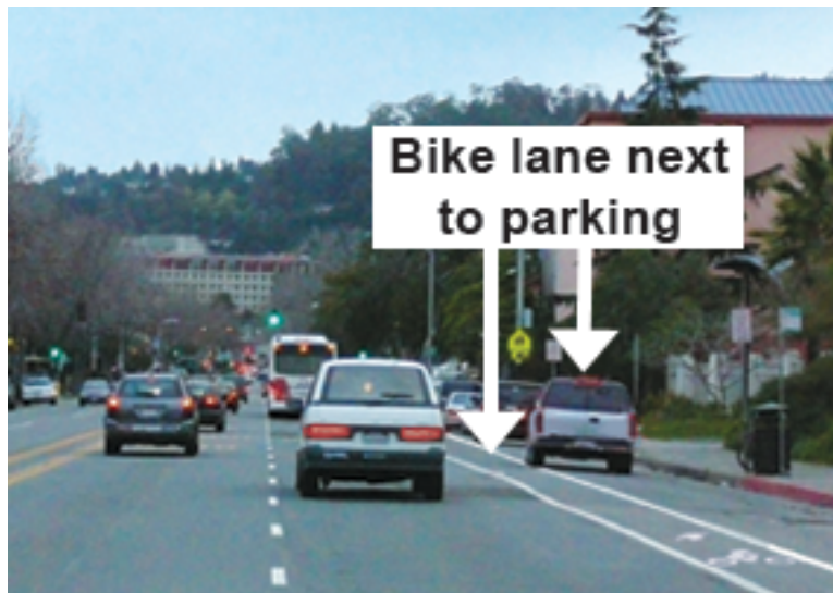
Figure 28. Striped bicycle lane next to on-street parking
