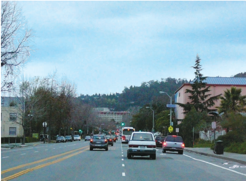
Figure 13. Commercial Street – Striped Bicycle Lane between Parking Lane and Curb
