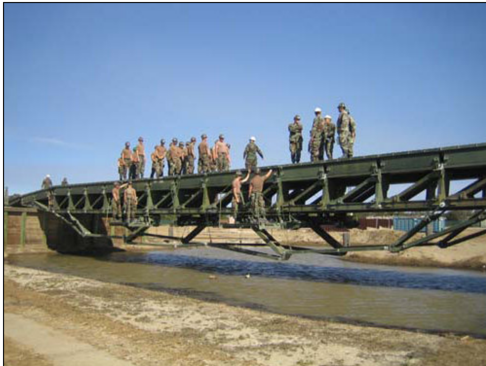
Figure 8-6 Photograph of MGB double-storey configuration with link reinforcement.
