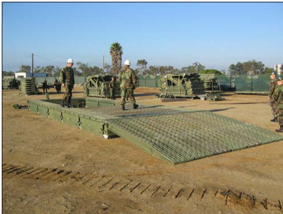
Figure 8-4 Photograph of MGB single-storey configuration.
