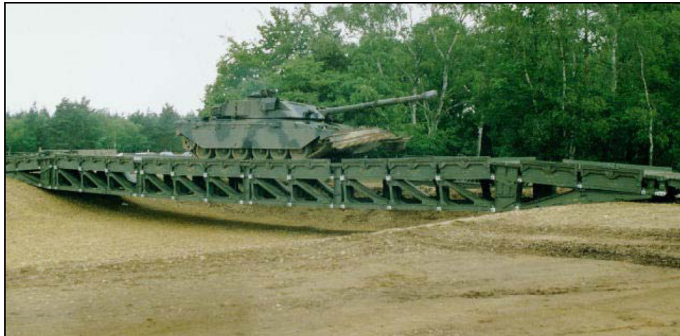
Figure 8-5 Photograph of MGB double-storey configuration.
