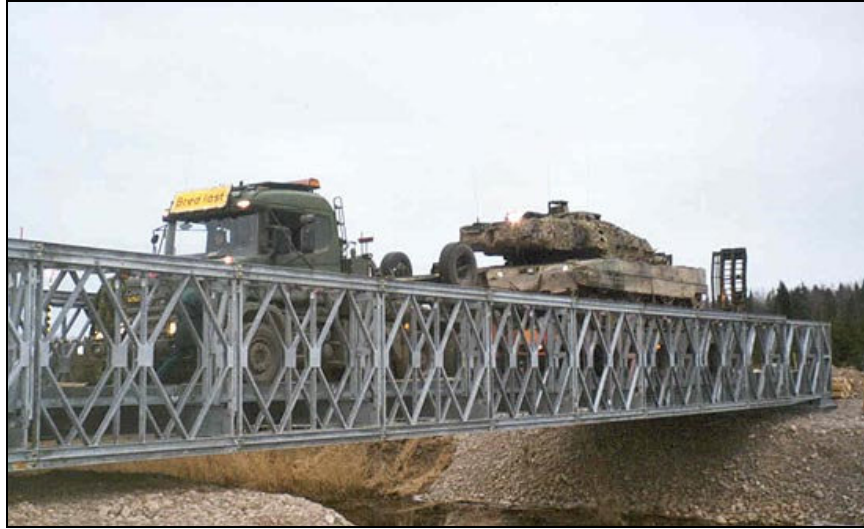
Figure 8-11 Photograph of the Mabey Johnson Bailey bridge.
