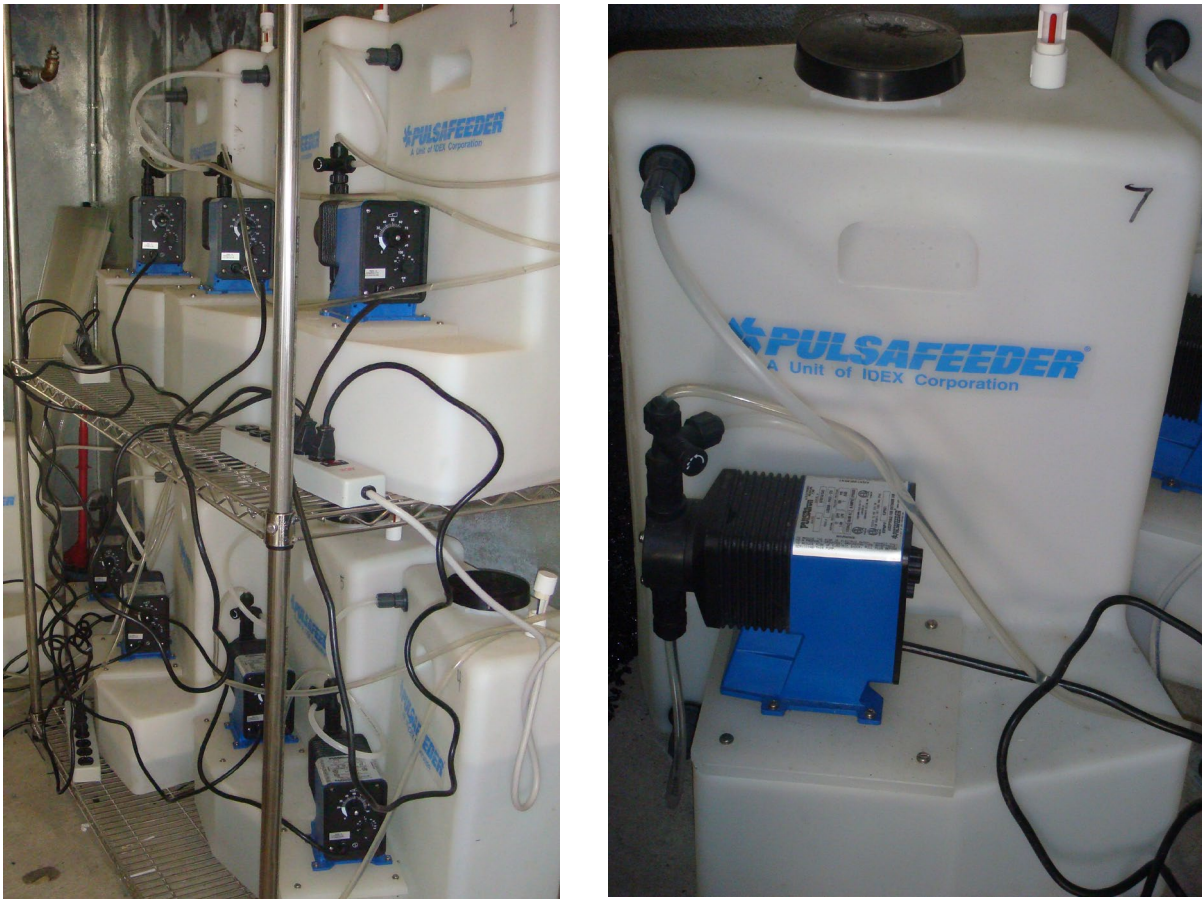
Figure 3-6 Variable speed pump attached to water storage tank and water delivery system
