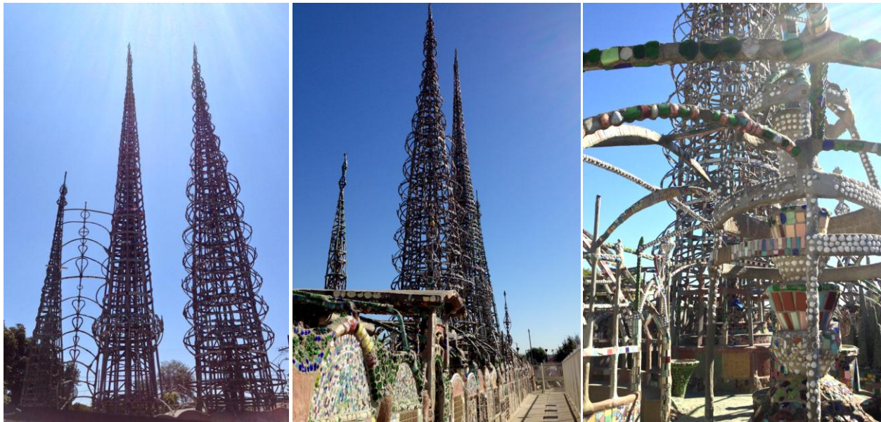
Figure 1.1: Photographs of the Watts Towers: A) view looking south, showing the three towers B) view looking east along the south wall C) view from inside the site, showing parts of the other structures and the overhead arches connecting all around the site
