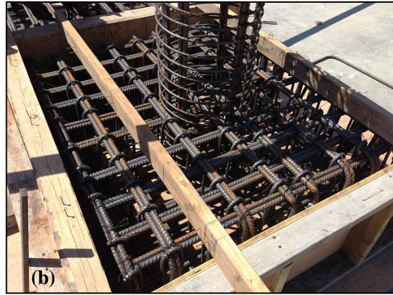
Figure 2. (a) Picture of the assembled aligned specimen and (b) reinforcing steel cage for the footing and the column.
