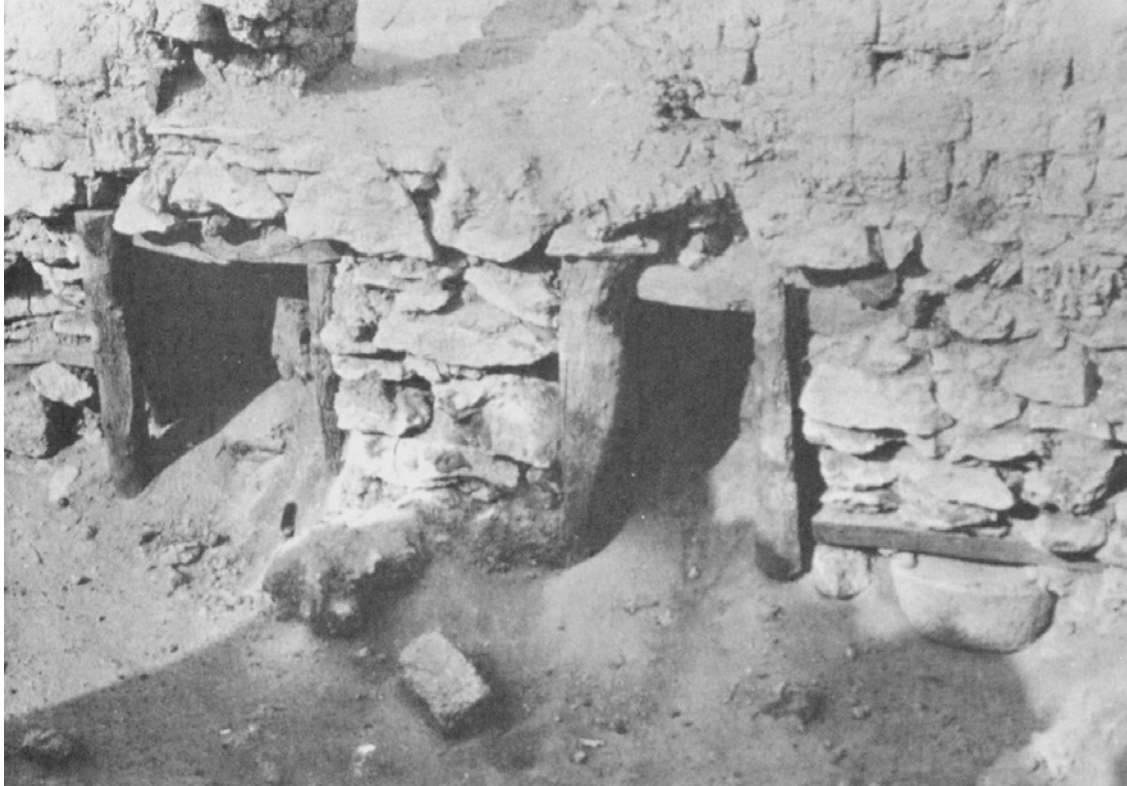
Figure 5.19. Animal pens from a Karanis courtyard, stone walls with wood reinforcement and a mudbrick plastered roof.
