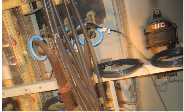
Figure 12: Typical installation of the split core current transducers on the left, the Rogowski coil CTs on the right.
