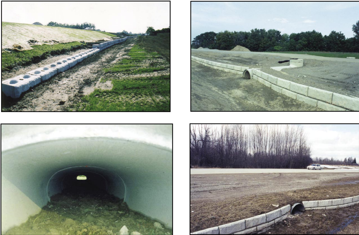
Figure 13. Bayview Avenue Extension–Examples of Amphibian Tunnel Construction, Interior, and Finished Look
