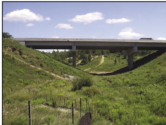
Figure 15. Landform Conservation–Three-span 81-meter Bridge
