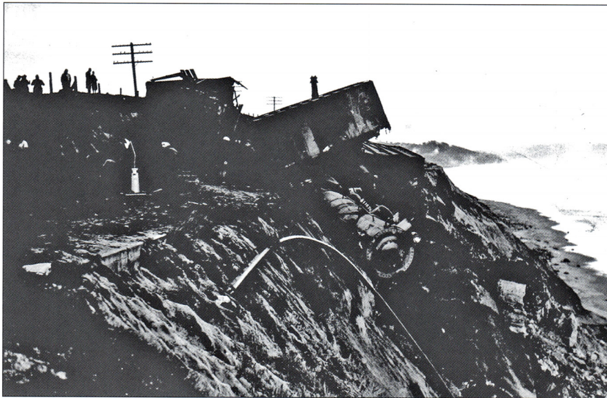
Figure 3. Train derailment in 1941 along the Del Mar seacliffs (photo courtesy of the Encinitas Historical Society).
