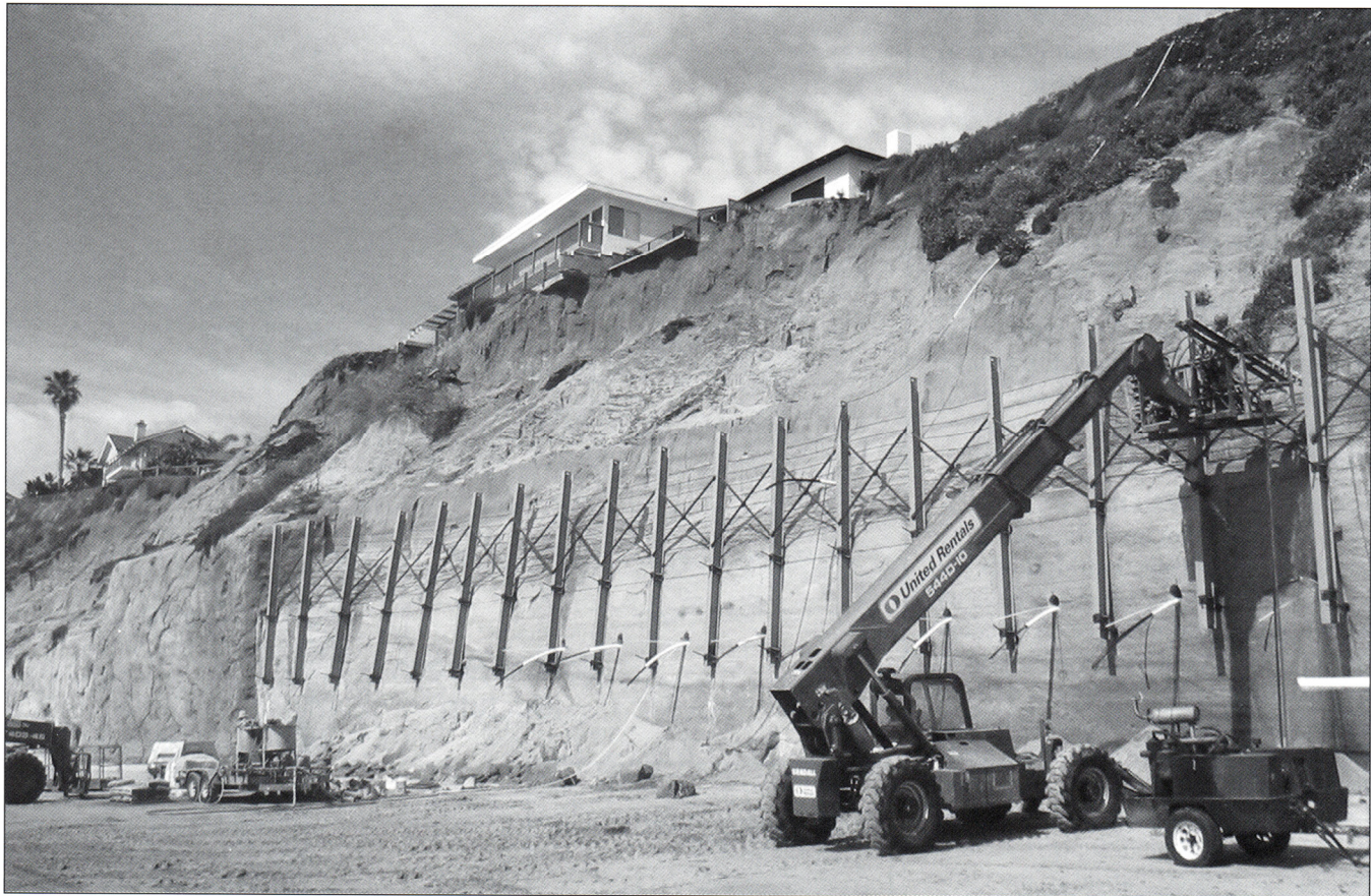
Figure 1. Construction of a tied-back artificial rock seawall in Solana Beach.
