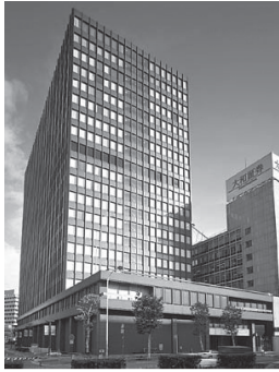
(c) Nippon Steel Building
