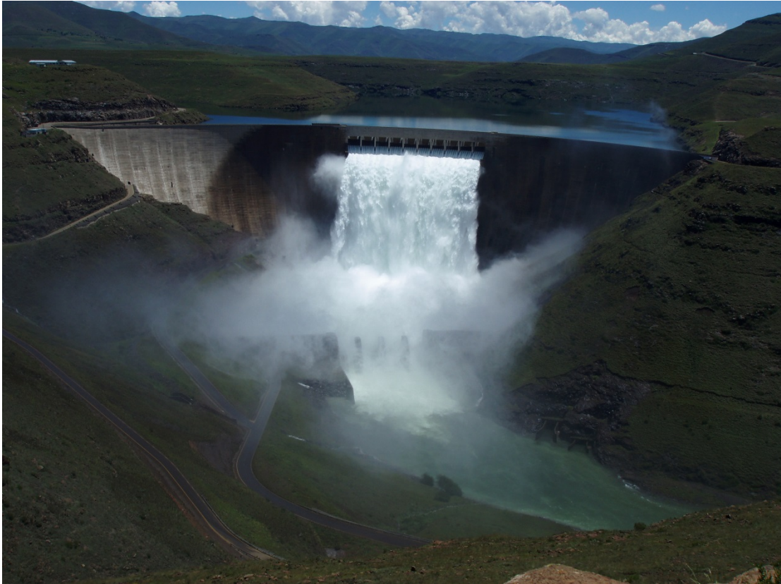
Figure 8: Katse Dam overflowing. Photo by the author.
