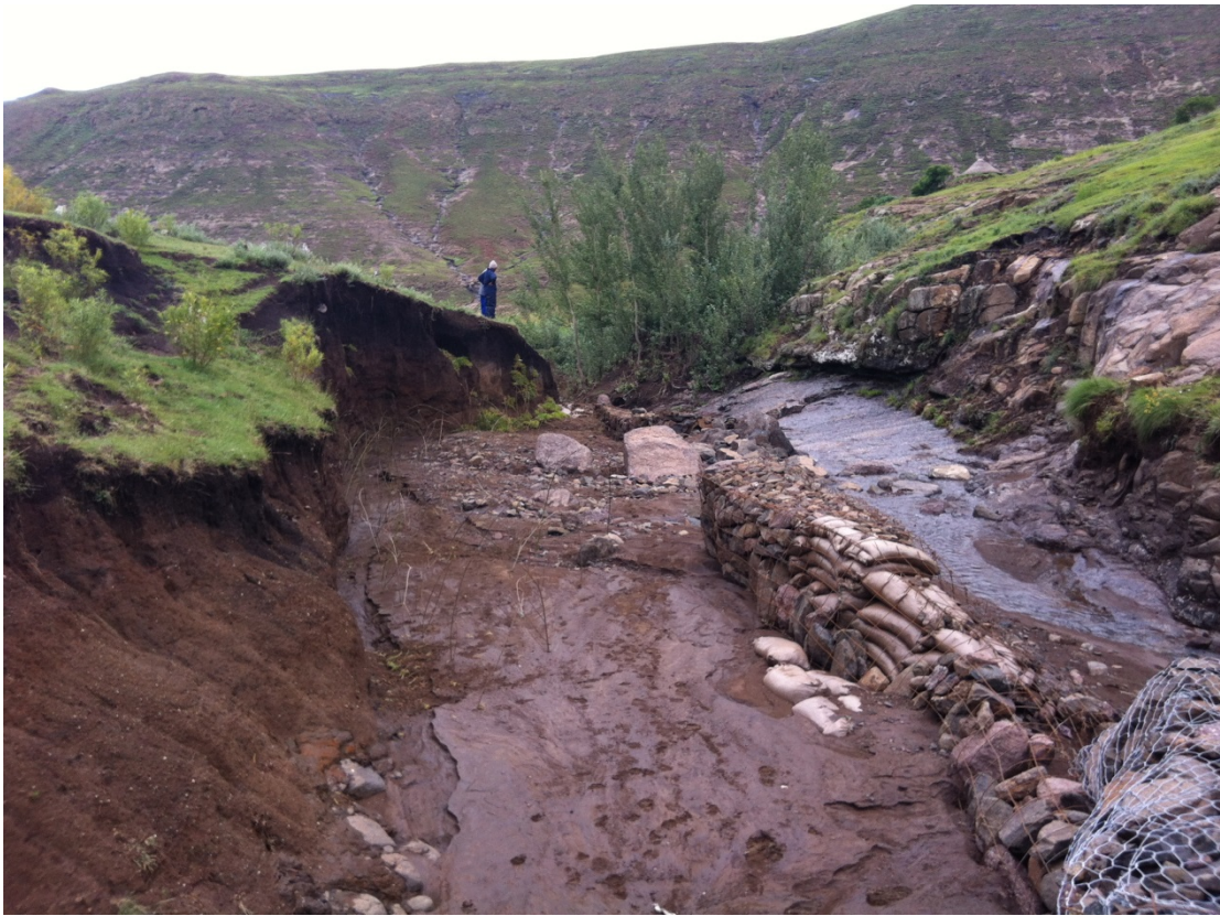
Figure 10: The gabions collapse at Khahleti and a cemetery washes away. Photo by the author.
