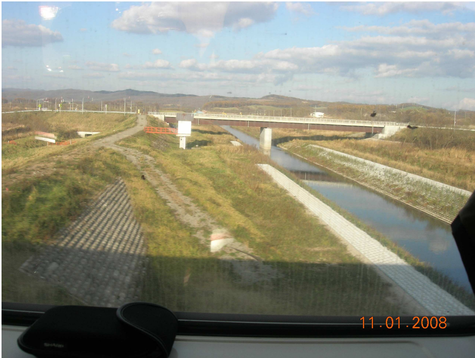
Figure 4: A Hokkaido “river improvement” project. Note the channelization, diking, and concrete banks. (Photo by author)
