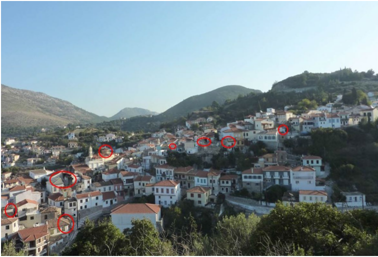
Fig. 25 Ano Vathy hill: Red circles denote damaged buildings. (Photo by Christos Giarlelis, HAEE/ETAM Team)
