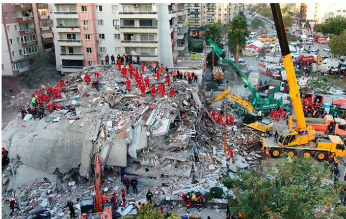
Fig. 15 Doganlar residential building, fully collapsed after the event (courtesy of Ali Aksoyer)
