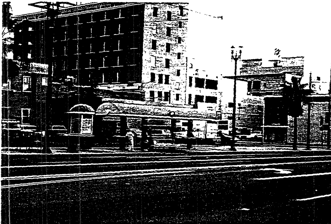
Photo Series 4.26 Pacific Ave. station: View of a bus stop at the east side of Pacific Ave. next to the station and, in the background, a multi-story building undergoing renovation.
