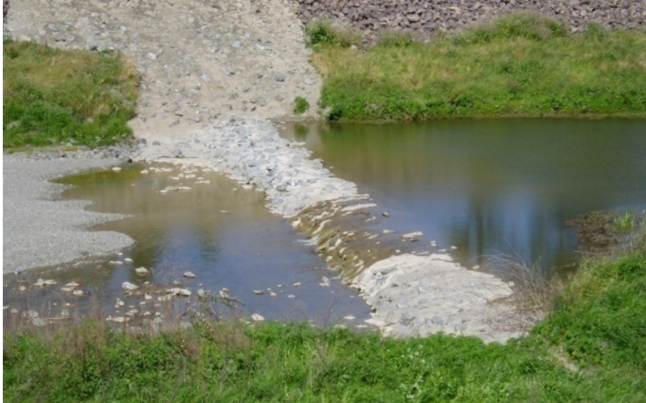
Figure 7. Photo of Check Dam #1
