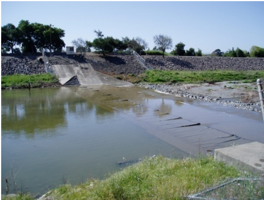
Figure 4. Photo of Rubber Dam #2
