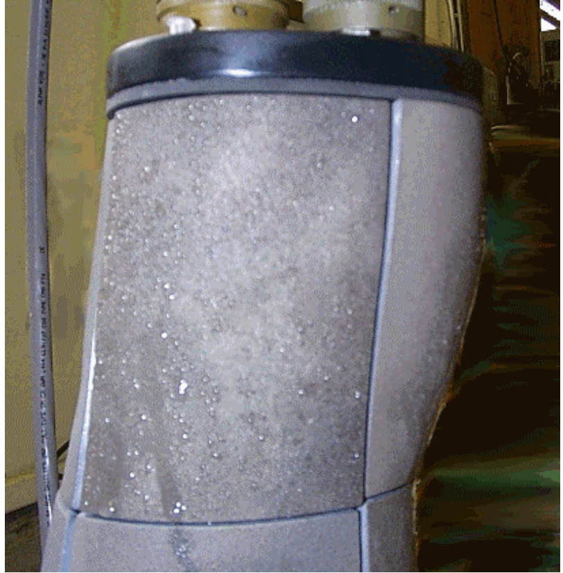
Figure 17: Surface Segment Sweating
