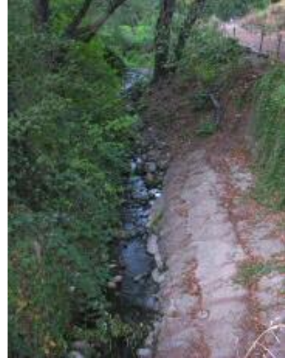
8b. View Upstream from Culvert (to the North)
