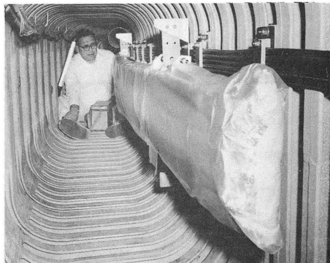
Installed quadrant cryopanel.
