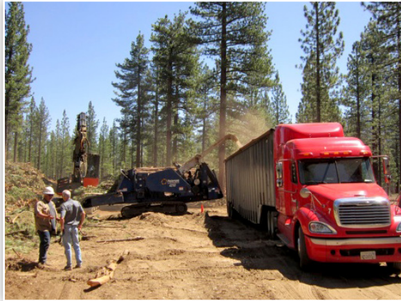
Left: Chip production for use at a biomass facility, Tahoe National Forest. Photo: B. Storey.
