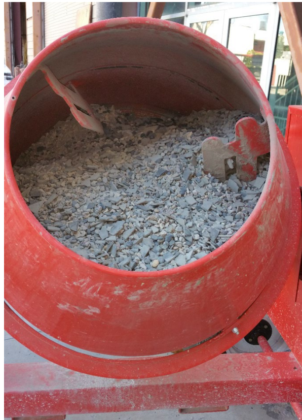
Figure 3.19. Sulfur concrete mix prior to melting.
