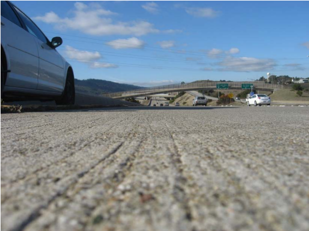
Figure A.7: Longitudinally broomed, OBSI=101.1 dB(A) (Section QP-146.3).
