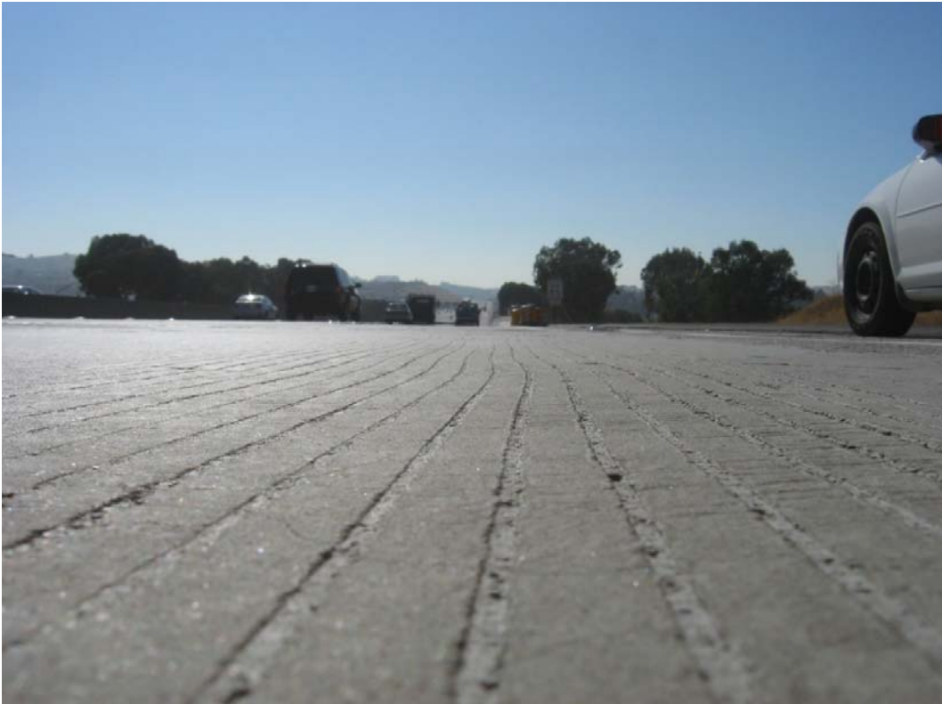
Figure A.9: Longitudinally tined, OBSI=102.7 dB(A) (Section QP-117.2).
