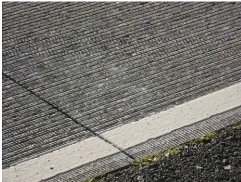
Texture and joint detail
