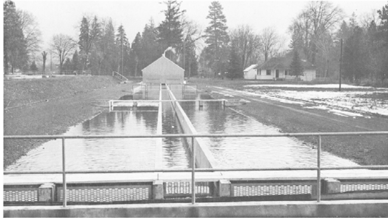
FIGURE 5. Modern brood pond and spawning house installation at Mt. Shasta Hatchery, Siskiyou County, California. Design permits fish to be moved into spawning house without taking them from the water. Photograph by George Farnham, February, 1958.
