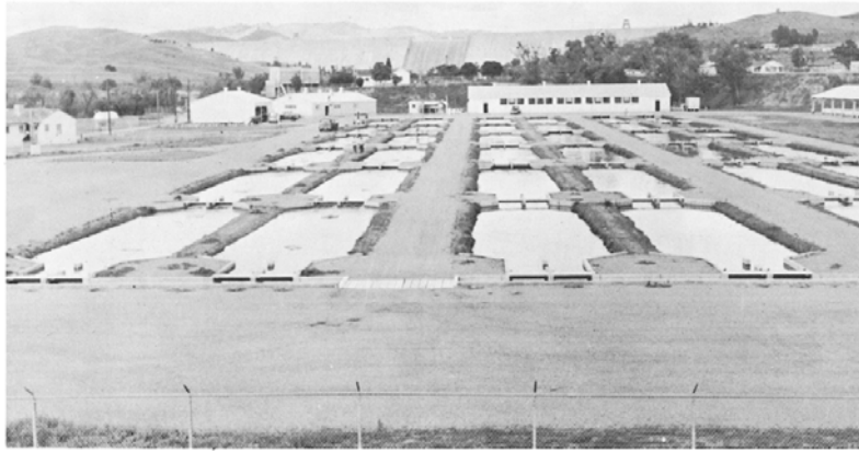
FIGURE 2. San Joaquin Hatchery, Fresno County, California. This hatchery is located below Friant Dam on the San Joaquin River and is operated on 25 c.f.s. of water received from Lake Millerton, a fluctuating reservoir behind the dam. This is an excellent example of a man-created hatchery water supply. To insure cool temperatures, water is drawn from a low level in the reservoir. This makes it necessary to treat the water by passing it through the aerating tower in left center of photo, which dissipates any harmful gases that may be present and adds sufficient oxygen to make the water safe for fish hatchery use. Photograph by William M. Carah, May, 1956.
