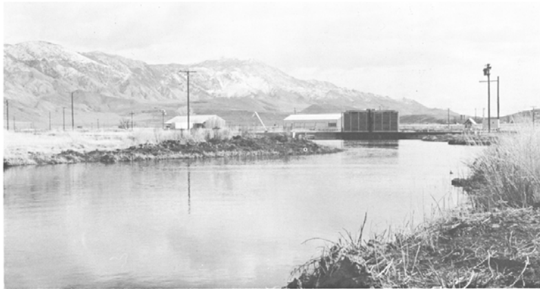
FIGURE 1. Fish Springs, Inyo County, California. A spring flowing approximately 20 c.f.s. of clear water at fairly constant temperature of 60 degrees F. provides this excellent hatchery water supply. In order to dissipate some harmful gases present and increase the oxygen content, a portion of the water used is treated by pumping it through the aerator in right center of picture. Photograph by Edwin P. Pister, April, 1958.
