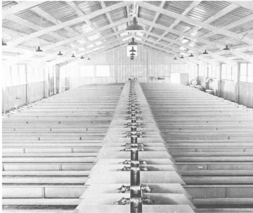
FIGURE 28. Aluminum hatchery troughs. Center water supply permits unobstructed aisle between troughs from one side of building to the other. Photograph by Harold Wolf, July, 1958.
