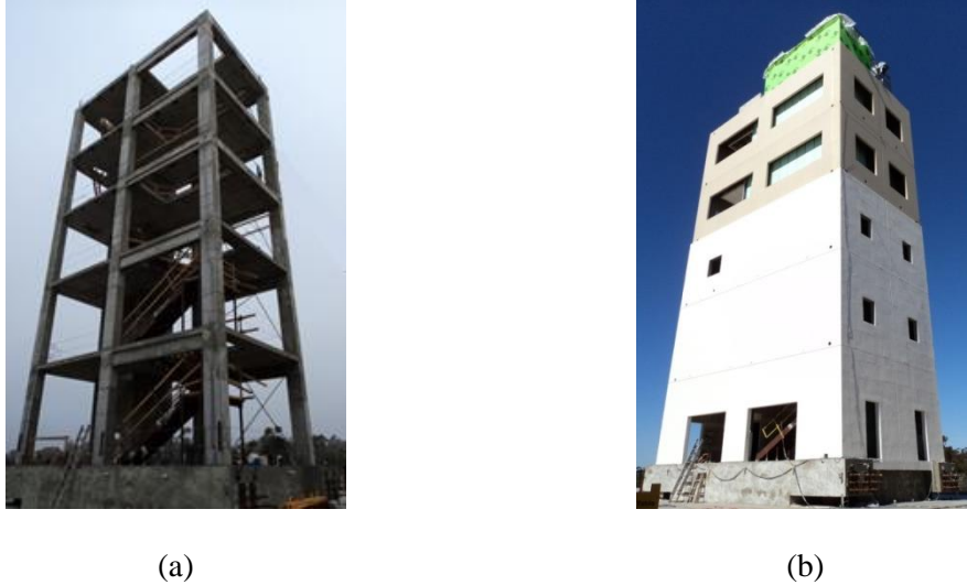
Figure 3.1: Views of the building specimen; (a) bare structure; (b) completed building.
