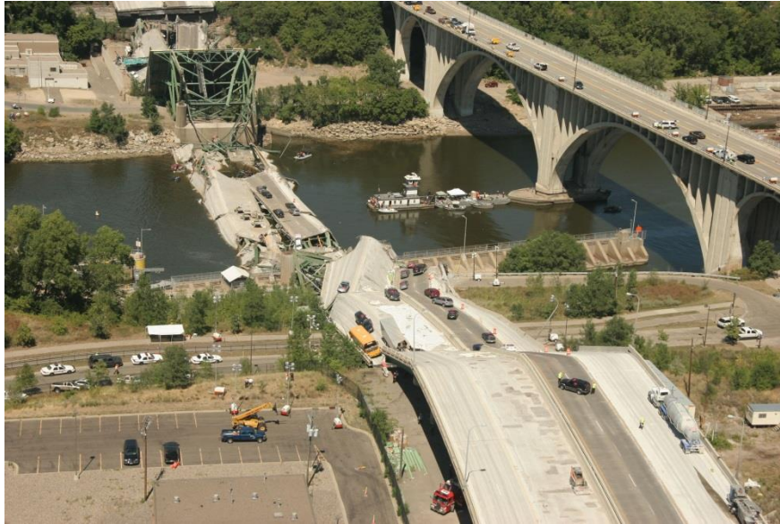
Figure 1.1: I-35W St. Anthony Bridge Collapse in Minnesota in 2007 (picture is taken from [2]).
