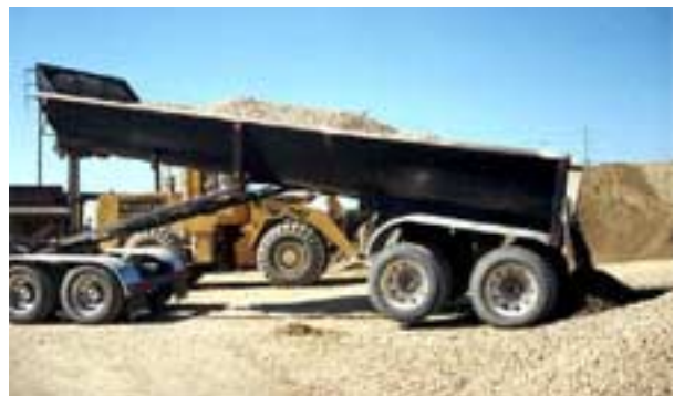
Figure 44. Delivery of aggregate with 22-ton capacity end dump truck.
