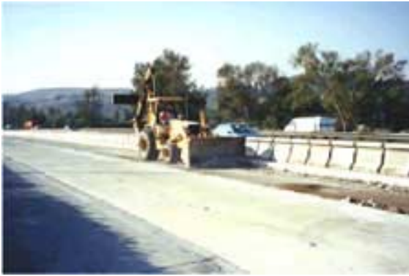
Figure 28. Cleanup of base with a small loader for “slab replacement” case.
