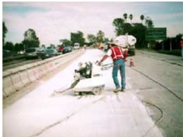
Figure 61. Sawing transverse and joints after 2 hours of curing.
