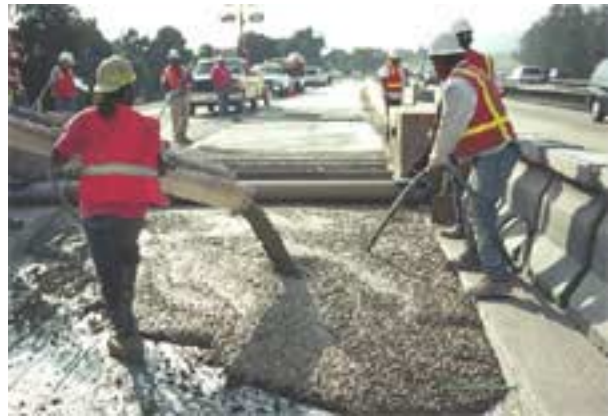
Figure 54. Example of good quality, fresh concrete.
