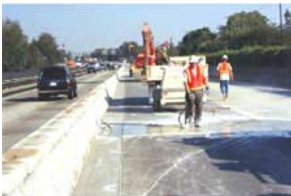
Figure 22. Breaking the starting point of the slab with a jackhammer.
