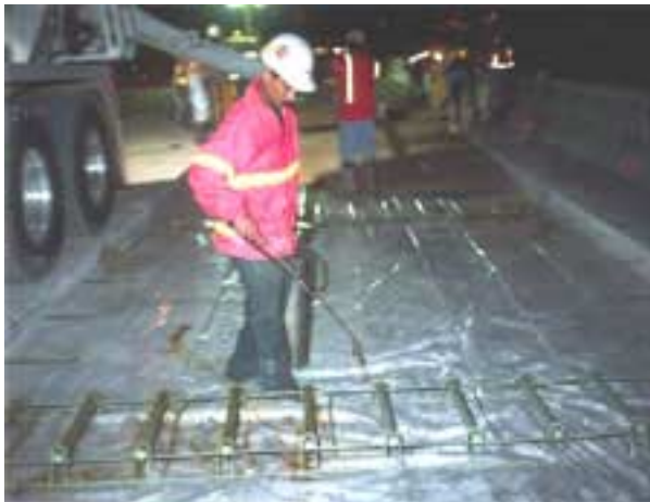
Figure 40. Application of release agent to the dowel bars..
