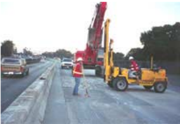
Figure 29. Impact demolition with a breaker for full depth replacement.
