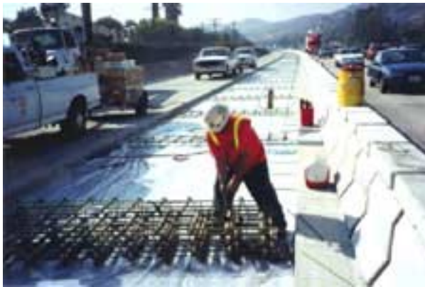
Figure 39. Installation of dowel bar basket.
