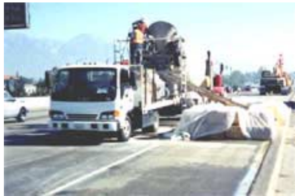
Figure 45. Temporary washing area for concrete buildup in the mixer drum.
