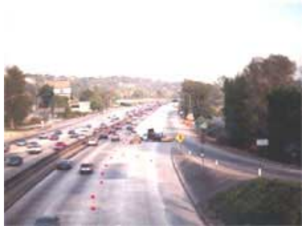
Figure 11. Beginning of closure of two right lanes with rubber cones.
