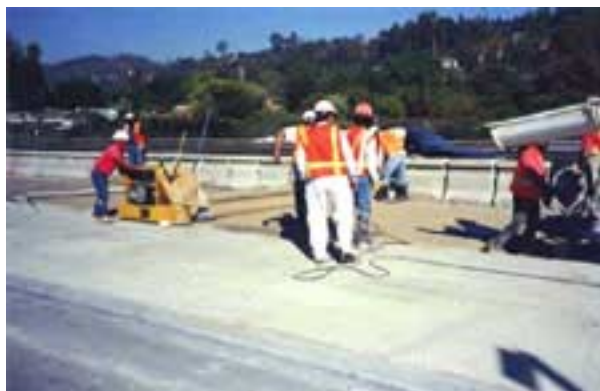
Figure 53. Manual alignment of the screed.
