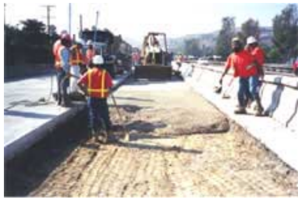
Figure 31. Placement of FSHCC CTB.
