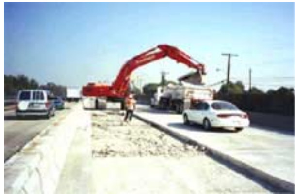
Figure 23. Non-impact demolition.
