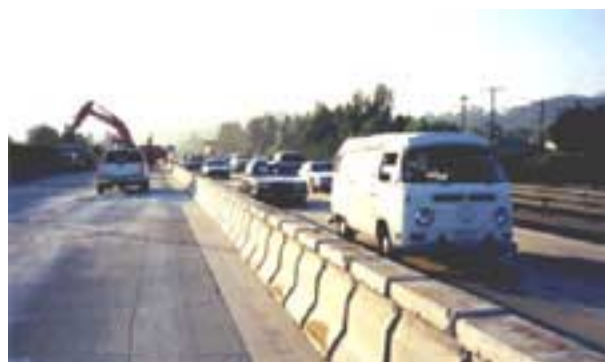
Figure 18. MCB installed as safety barrier during the weekend closure.
