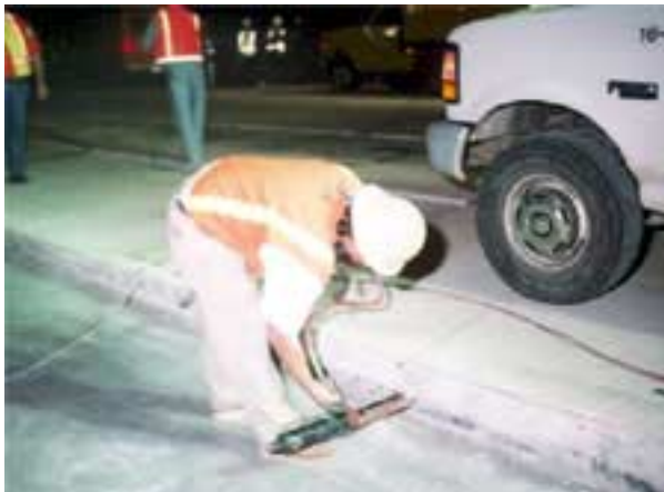
Figure 37. Injection of epoxy into the bar holes.
