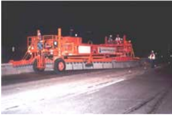
Figure 19. Installation MCB using transfer and transport machine.
