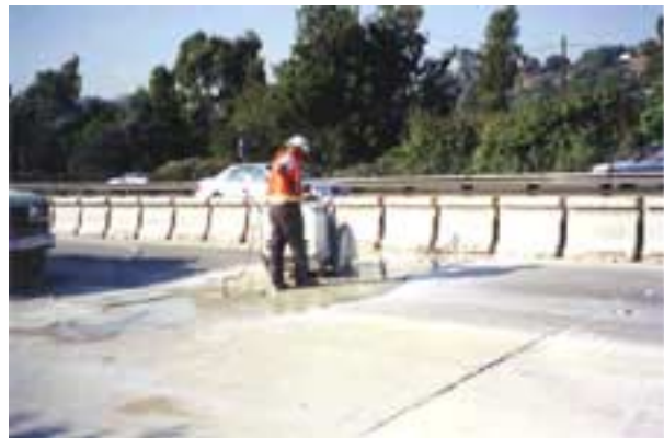
Figure 20. Slab cutting for non-impact demolition method.
