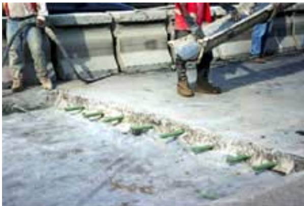
Figure 41. Placement of dowel bars in existing slab.
