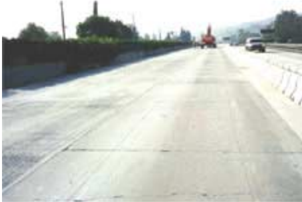
Figure 21. Slab panels cut into three pieces longitudinally.
