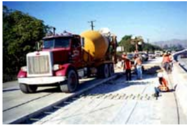
Figure 47. Concrete discharge and paving operation.
