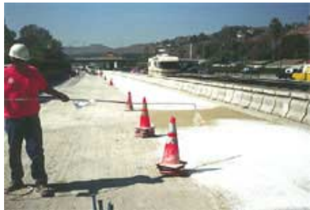
Figure 60. Curing compound being applied manually.
