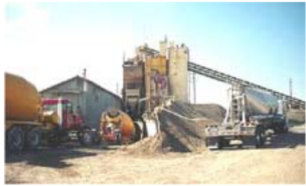
Figure 42. Western Rock batch plant, 220 m 3 per hour capacity.
