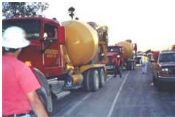
Figure 48. Queuing of mixer trucks waiting to discharge during screed breakdown.
