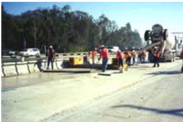
Figure 59. Manual finishing and texturing of the pavement.
