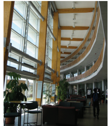
The atrium provides a thermal buffer for the north-facing offices
