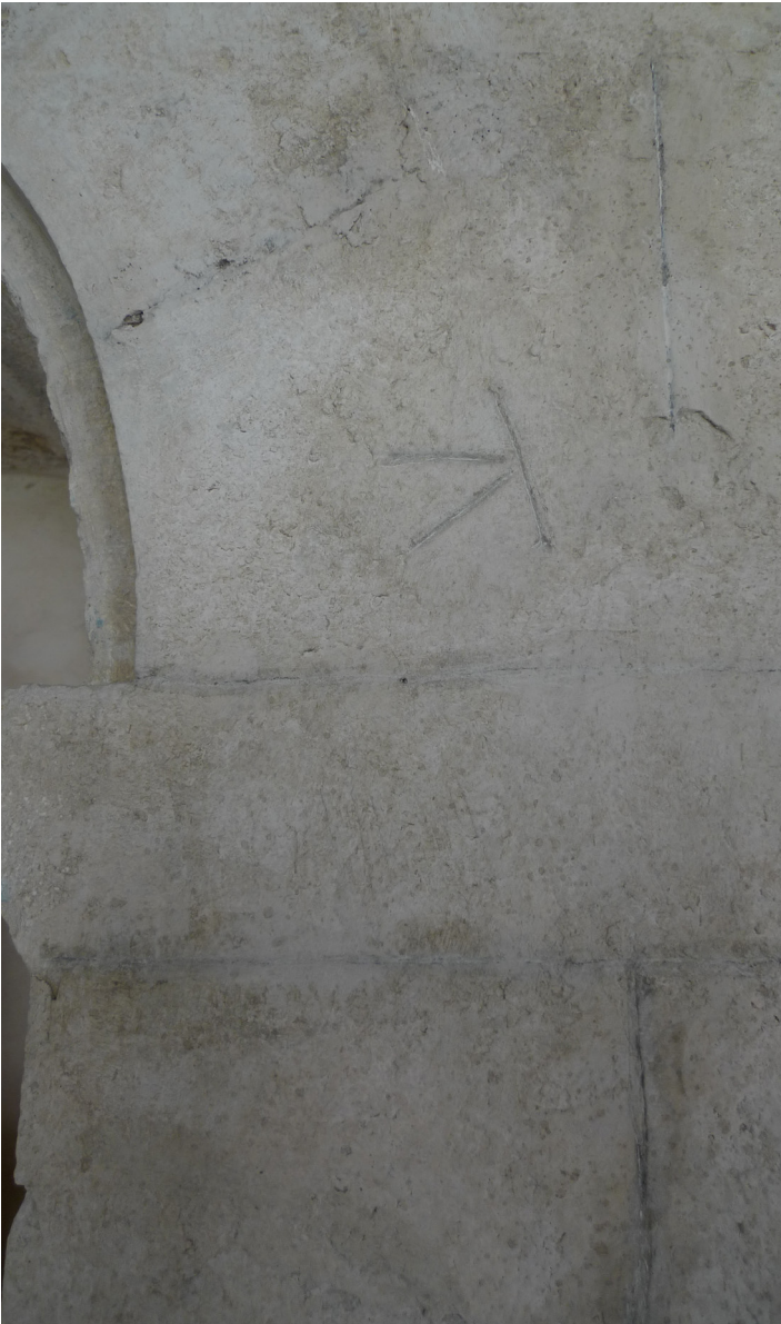
Figure 1 Signature stones near an arched opening in the Abbaye de Notre-Dame de Sénanque (founded 1148). Photograph by author.
