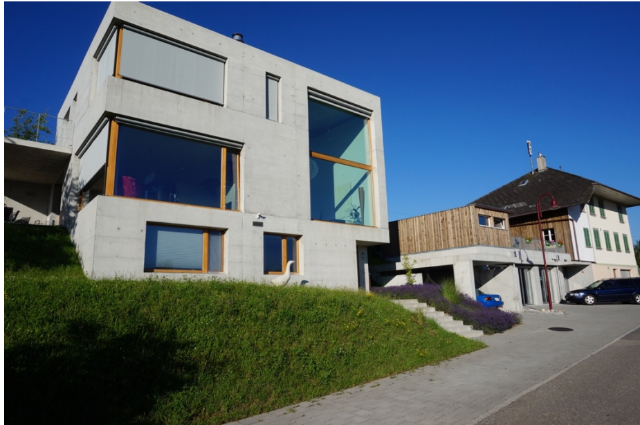
Image 9: Worb, Switzerland, schoolhouse next to modern apartments, July 2014
