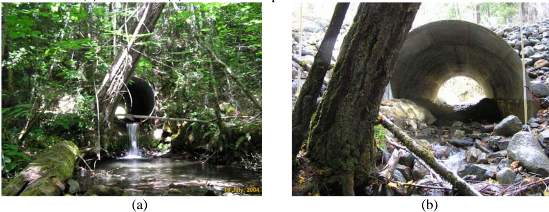
Figure 3. Example of fish-passage improvement and reduction in risk of catastrophic failure at Stanza Creek (a) before and (b) after culvert replacement.
