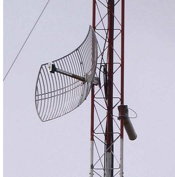
Figure 5: A parabolic and yagi antenna on top of a tower at UNAM. A splitter is connected to the wireless card to attach two antennas to the same antennae
