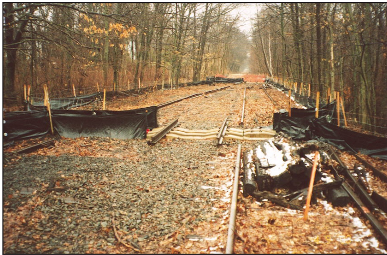
Photo 2. Silt fencing as surrogate barrier fence in the project area. Woodlot Alternatives, 2003.
