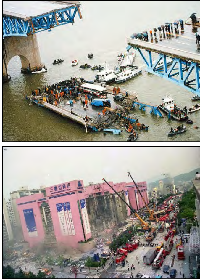
Figures 7a (top). Collapse of the Söngsu Bridge (1994). Source: Yonhap News Agency. Figure 7b (bottom). Collapse of the Samp'ung store (1995). Source: Yonhap News Agency.
