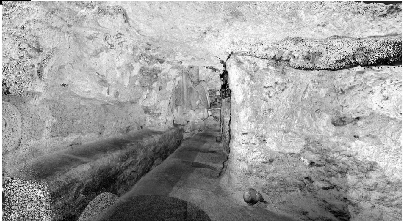
FIGURE 10. Still image of the interior of the Lidar model of Str. M7-1. The architectural step that connects the two masks of the Accession Platform is clearly visible on the left side of the image. Two of the tracking balls used to stitch the Lidar scans together are visible on the floor.
