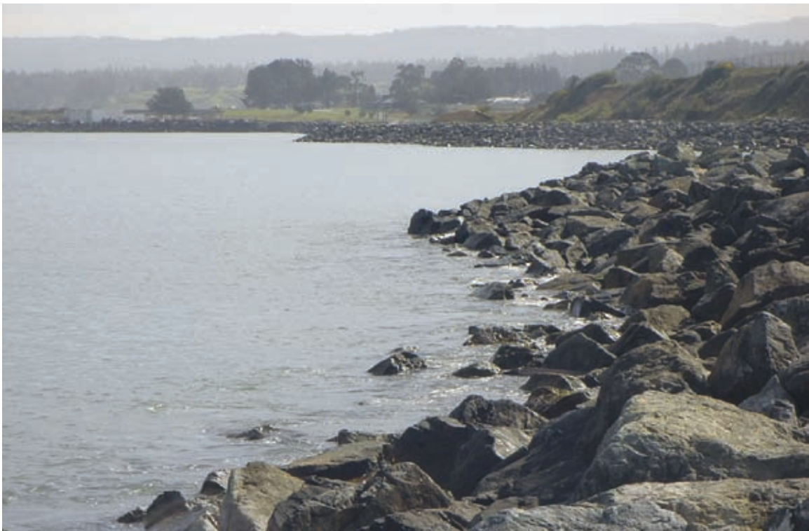
Figure 3. The shore of Entrance Bay of Humboldt Bay, Humboldt County, California, is lined with rip-rap due to increased wave action. This photo was taken near the town of King Salmon, along the eastern shore of Entrance Bay.
