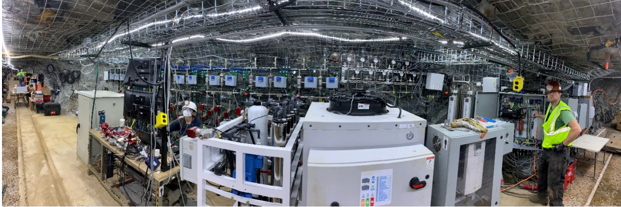
Figure 16: Panoramic of the system as installed on the 4100 level. Note the modular plumbing hung on the wall behind the other equipment and the control computer.
