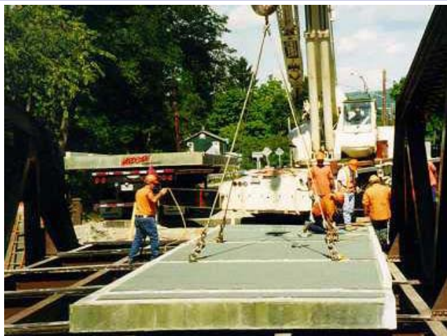
Figure 37: Installation of all-composite bridge deck of NY 367 over Bentley Creek, Chemung County, New York, USA.
