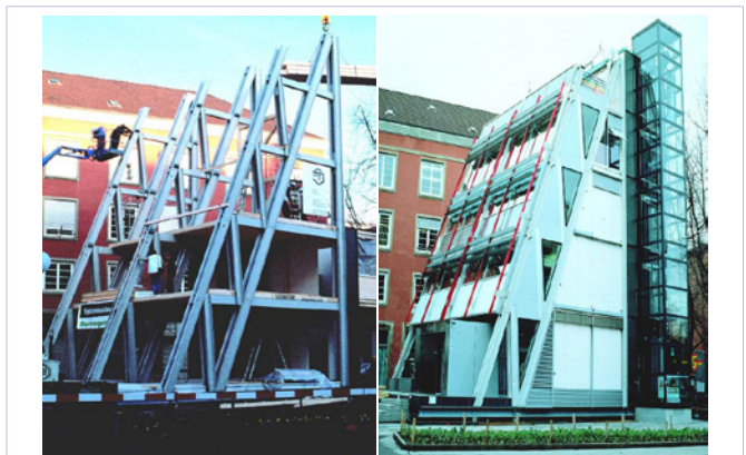
Figure 31: The eye catcher pultruded building during and after construction.
