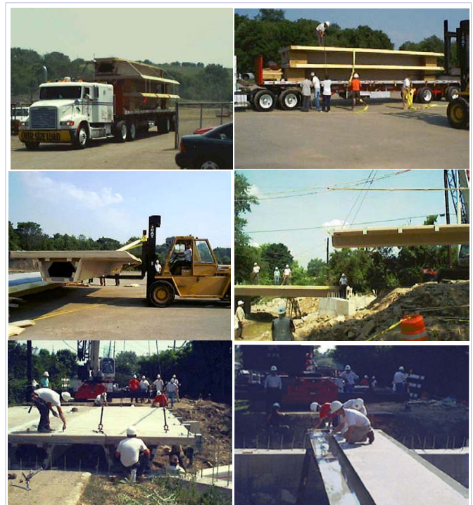
Figure 40: Construction stages of the smith road bridge all-composites bridge, Ohio, USA.
