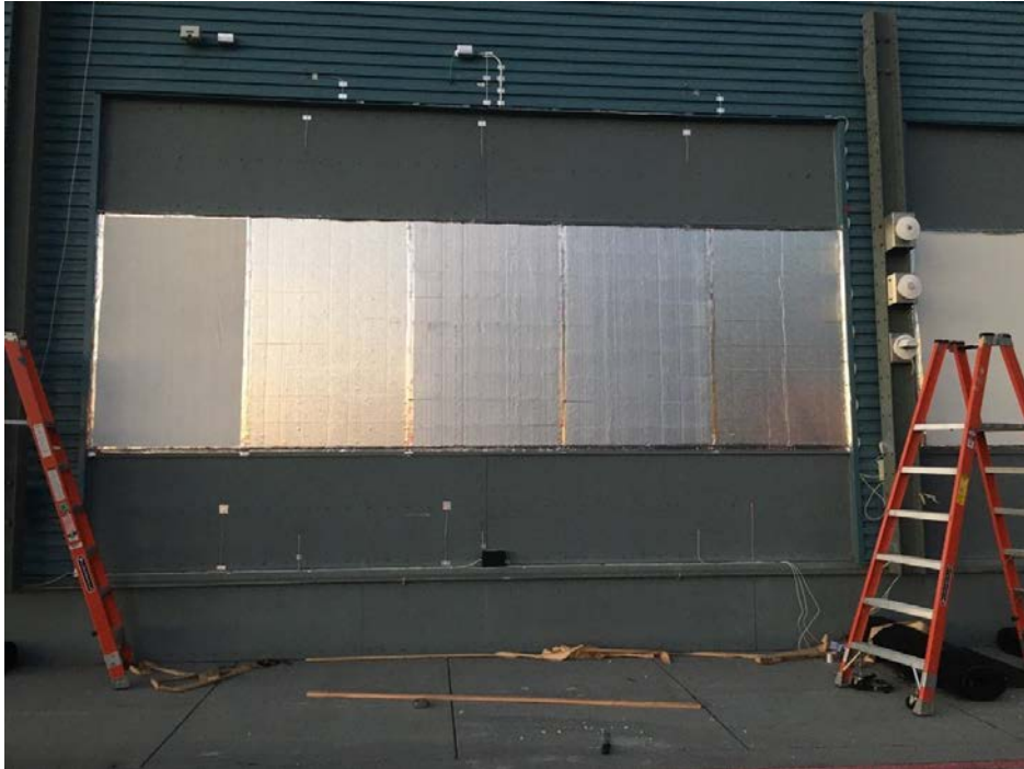
Figure S1. Foam panels on exterior of windows during Conference experiments.
