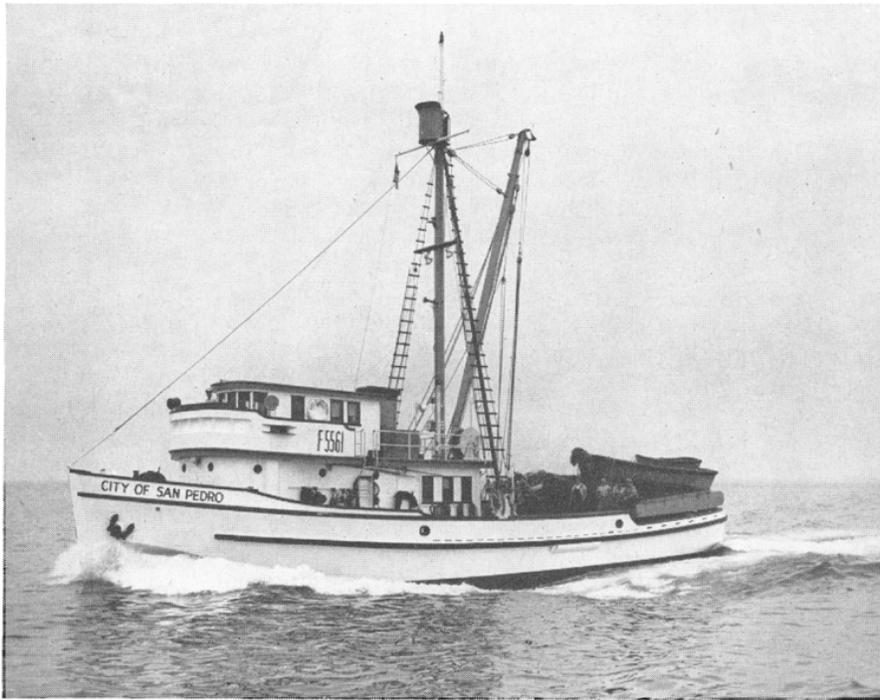
FIGURE 97. A representative of the modern purse seine fleet. These vessels fish seasonally for sardines, mackerel and tuna. The larger ones are depending increasingly on tuna and are, therefore, adapting their refrigeration plants to carry part of their load in brine. Photographed by Kent Hitchcock, Balboa, California, 1947
