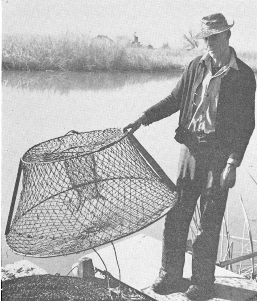
**FIGURE 25.** A carp fisherman with a new type of carp trap, Seven Mile Slough, near the mouth of the Mokelumne River. Rolled barley is tied, in fine-mesh sacks, near the funnel-shaped entrance for bait. Fishermen sometimes fish with 50 of these traps at one time, and they have caught as much as 3,500 pounds of carp in two days of fishing. Photograph by Felix A. Miller, December, 1948
