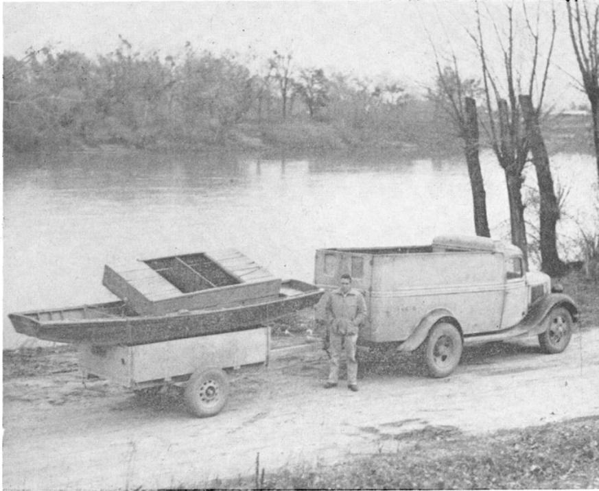
**FIGURE 26.** A rough fish fisherman's equipment, Sacramento River near Broderick. The tank truck is equipped to haul live fish to the markets. The trailer holds the seine, a skiff and a live box, used to keep the fish alive during fishing operations. Photograph by Felix A. Miller, December, 1948
