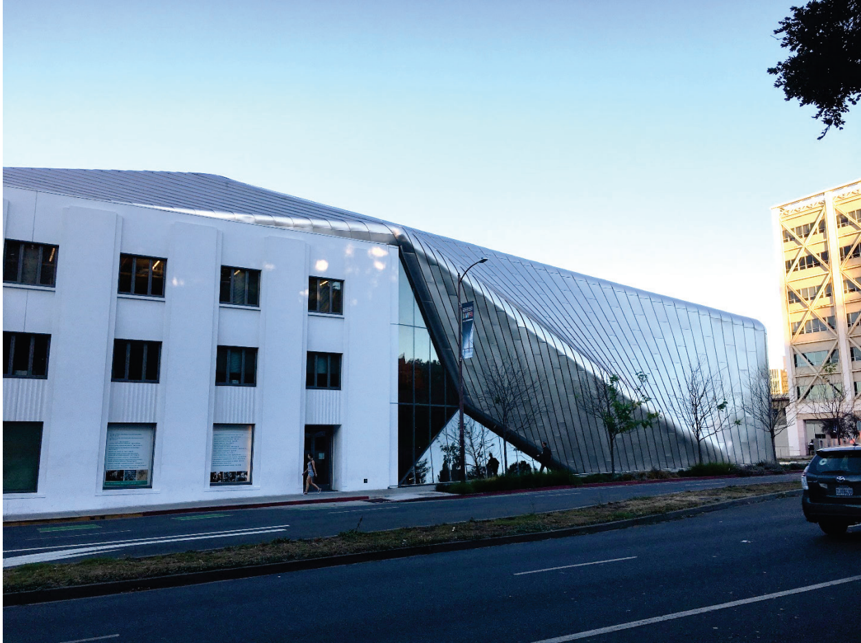
Figure 6. White wall (left) and bare stainless-steel wall (right) on the Berkeley Art Museum and Pacific Film Archive in Berkeley, CA.
