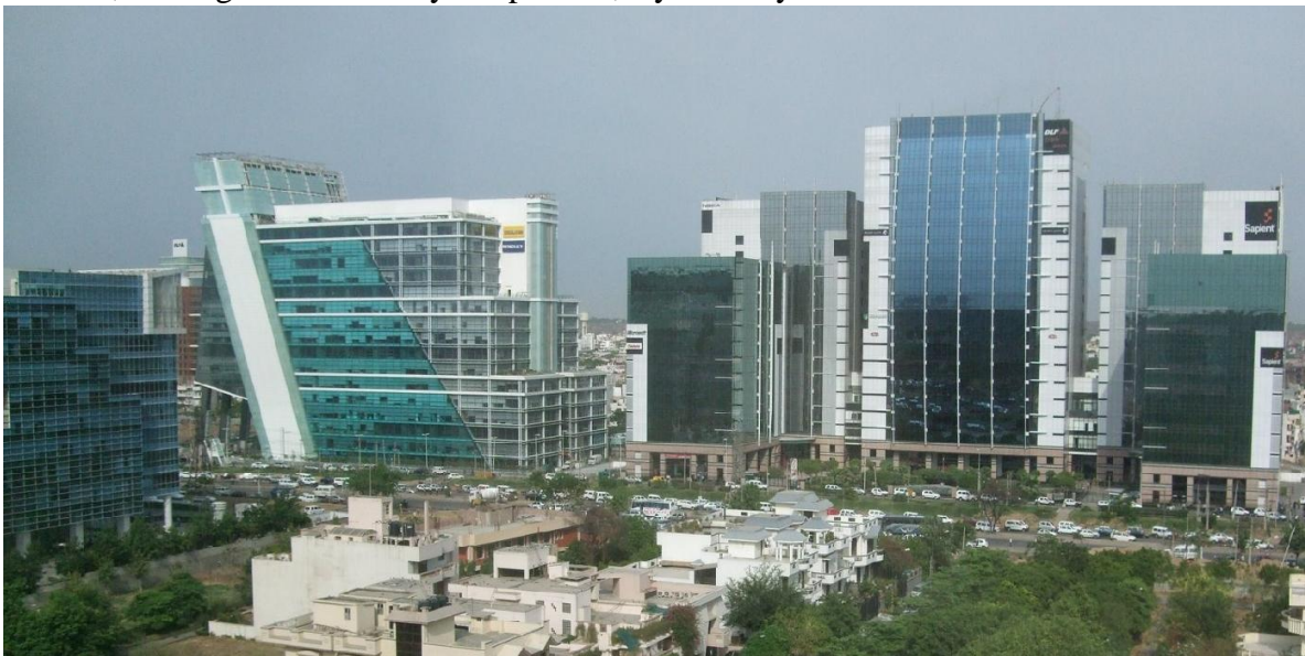
Figure 3.4: Newer, multistory glass and steel construction being built in Gurgaon, Haryana. Image courtesy of the Free State Initiative ( http://freestateinitiative.org/gurgaon-the-singapore-of-india ).
