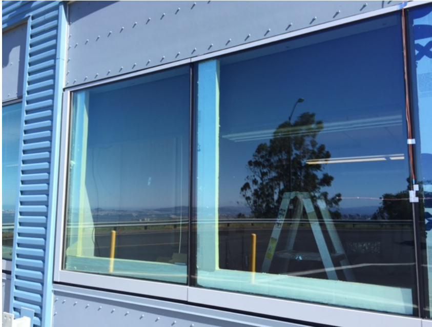
Figure 4. Foamcore panels were used to test smaller window-to-wall ratio.
