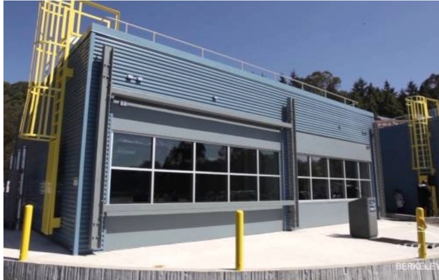
Figure 3. External view of the FLEXLAB rotating testbed
