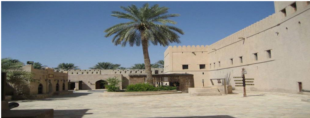
Figure 3.1 Inside the Nizwa fort. The palm constructed 'arish may be seen on the far side by the exhibit area, formerly the old prison
