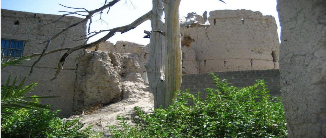
Figure 3.0 Crumbling ruins of houses and watch towers in the oldest residential quarter of the city, harat al aqr
