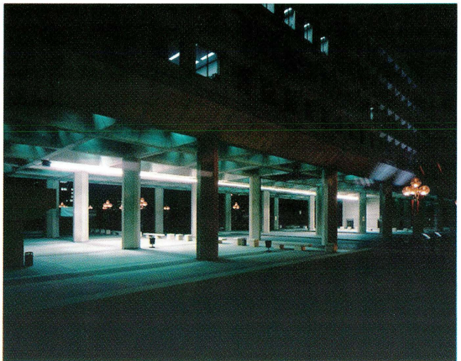
Figure 3. A photograph of DOE's Forrestal Building showing the 240-ft.-long light pipe running over the plaza. The enclosure that houses one of the two high-power sulfur lamps is just visible at the left end of the light pipe. The old lighting system, consisting of 280 mercury vapor fixtures, was also switched on for this photograph but is ordinarily off.
