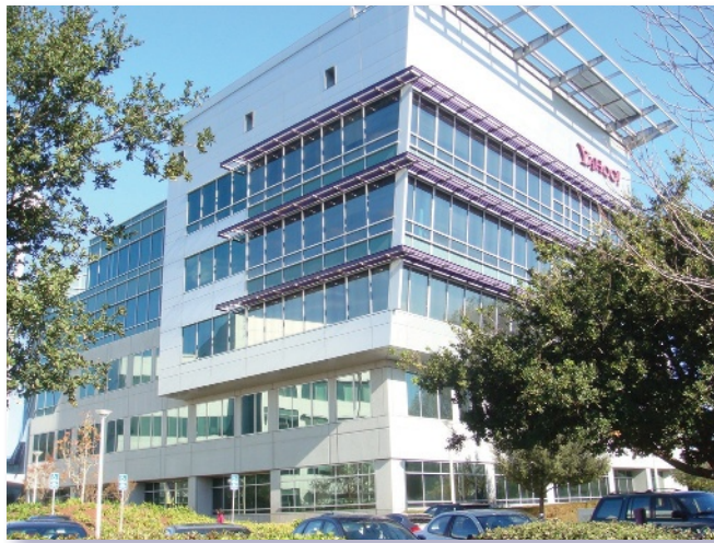
FIGURE 1 Yahoo! Buildings. Typical facade, floor plan (orange indicates open office), and open plan office interior.
