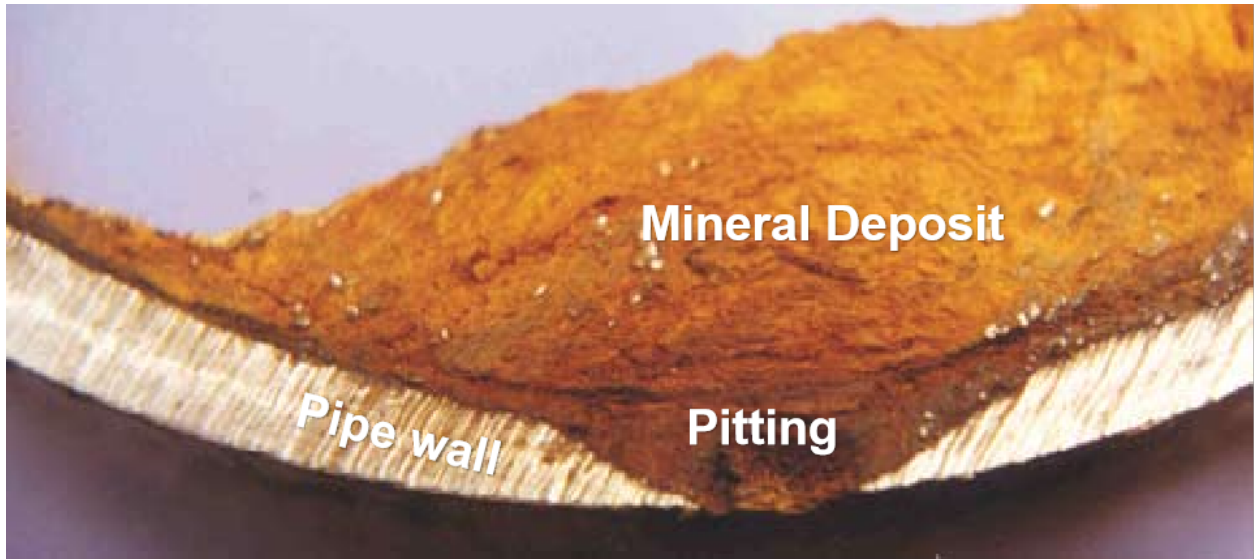
Figure 1.1: Photograph of a sectioned mild steel pipe that failed in service at Three Mile Island Nuclear Power Station.
