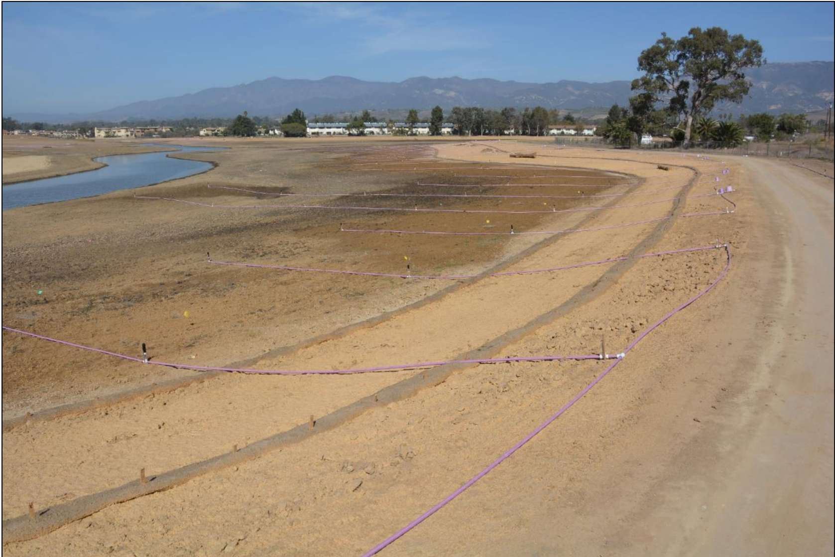
Baseline photo – post-grading, October 10, 2017.
