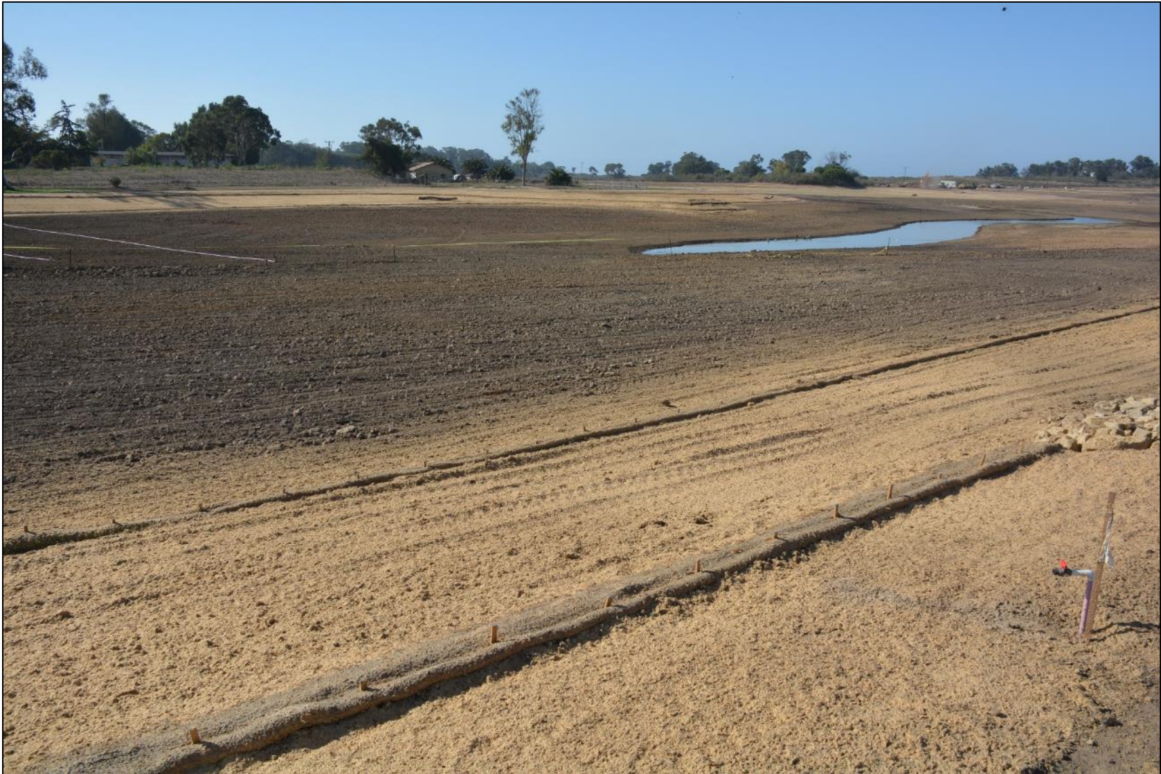
Baseline photo – post-grading, October 10, 2017.
