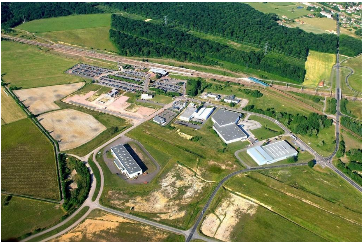
Figure 3. The Coriolis business park in 2012.
