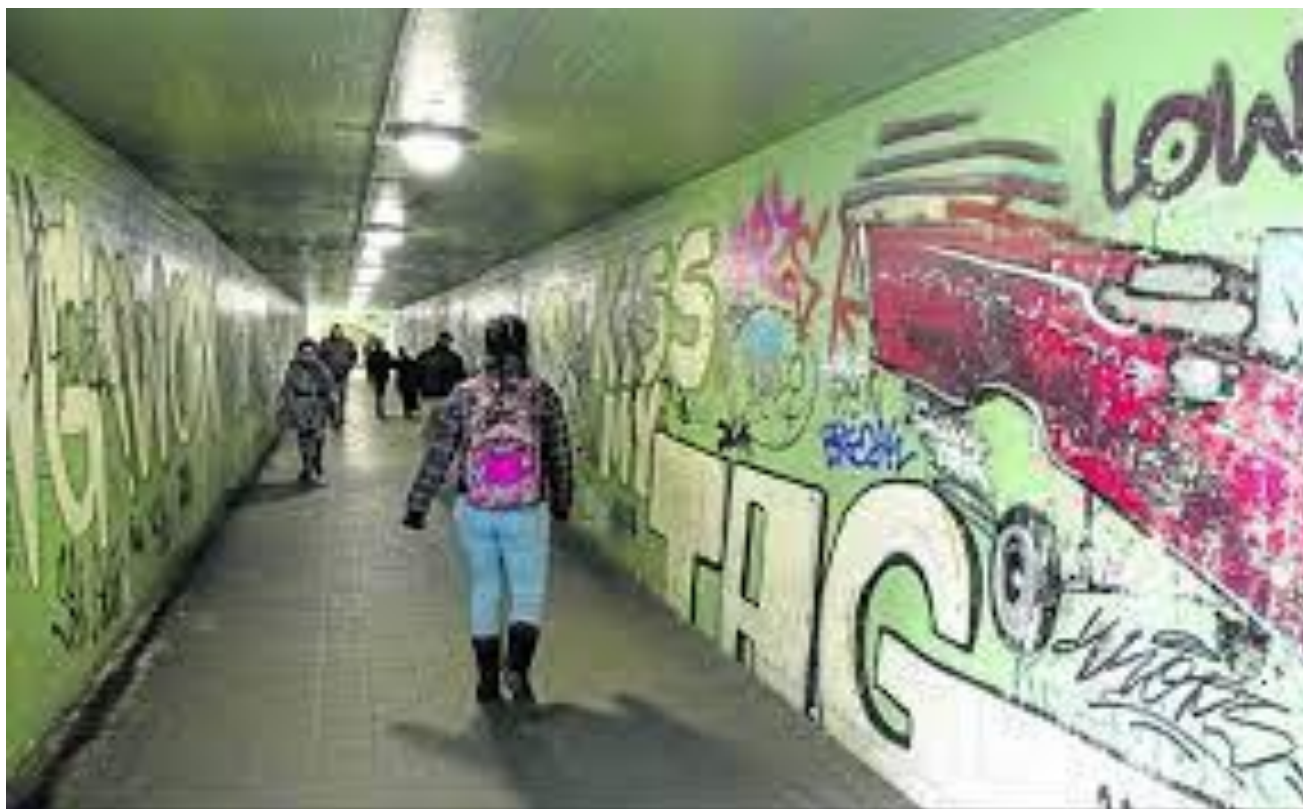
Figure 27. Pedestrian tunnel in Valladolid.
