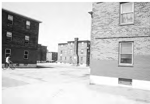
West Broadway, buildings not renovated in first phase of project
