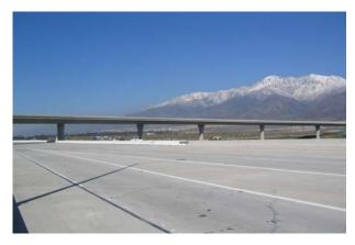
The overall objective of the study was to assess Caltrans long-life pavement rehabilitation strategies for rigid pavements, which aim to add at least 30 years of service life, require minimal maintenance (although zero maintenance is not a stated objective), and allow approximately six lane-kilometers to be rehabilitated or reconstructed within a construction window of 67 hours.
