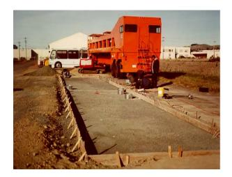
The concrete test sections constructed at the Richmond Field Station (RFS) demonstrated that instrumentation could be successfully embedded in the concrete. The methodologies used to place the instruments were considered adequate given that all gauges functioned correctly throughout the entire test program. The instrumentation and placement methods were developed with help from the US Army Corps of Engineers, Minnesota DOT, and Ohio University.
