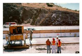
Construction of the fast-setting hydraulic cement concrete (FSHCC) test sections in Palmdale was completed in mid-1998 with the successful installation of all instrumentation for later modeling. The contractor selected a blend of 80 percent FSHCC and 20 percent Type I/II portland cement to meet the FSHCC specifications. The South Tangent concrete placement took two days while the North Tangent took three days. Early setting of the concrete in the haul
