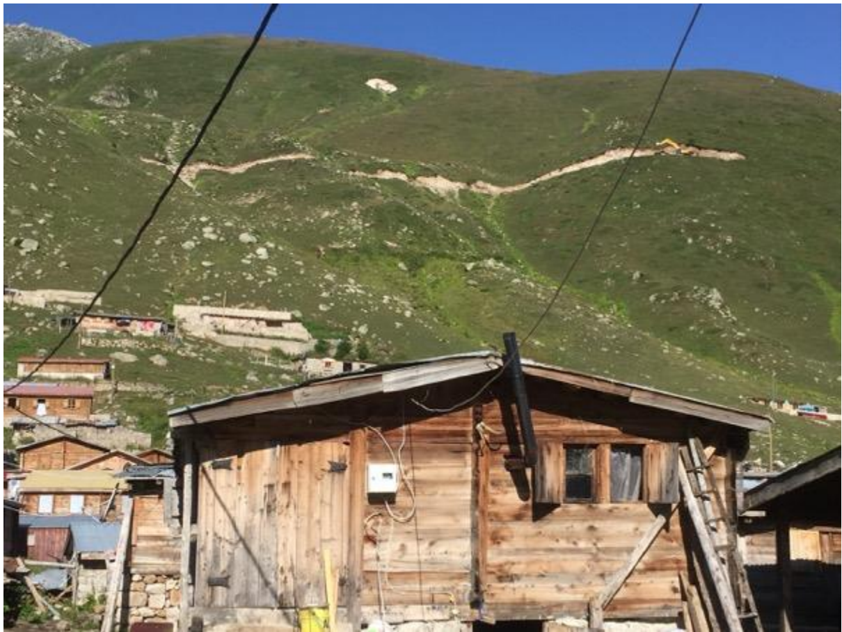
Figure 5.2: A bulldozer opening the “Green Road” in the mountain behind villagers’ houses. Kavrun Plateau, Çamlıhemşin, Rize. © Sevi Bayraktar, 8.1.2017.
